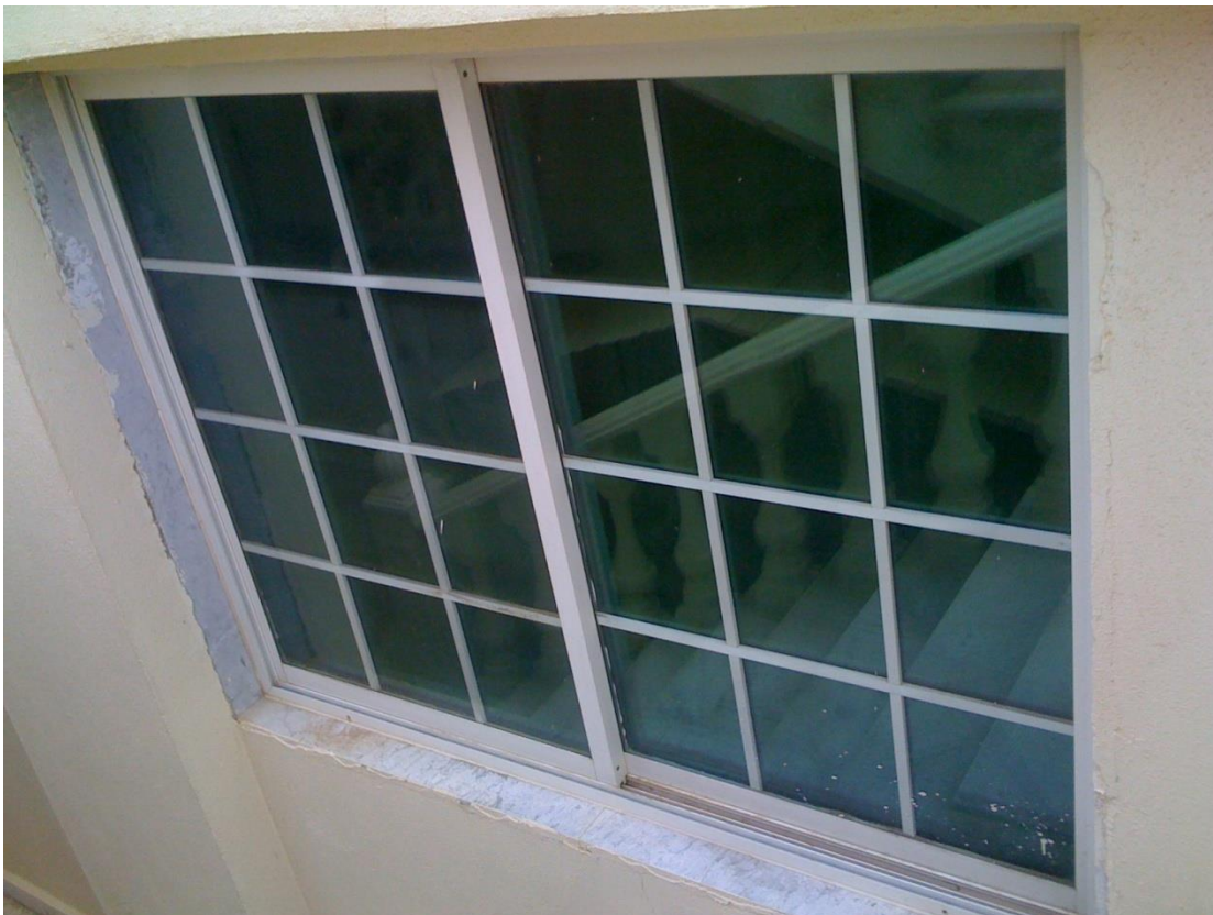
Picture 7: totally shaded window facing east (Basement).
